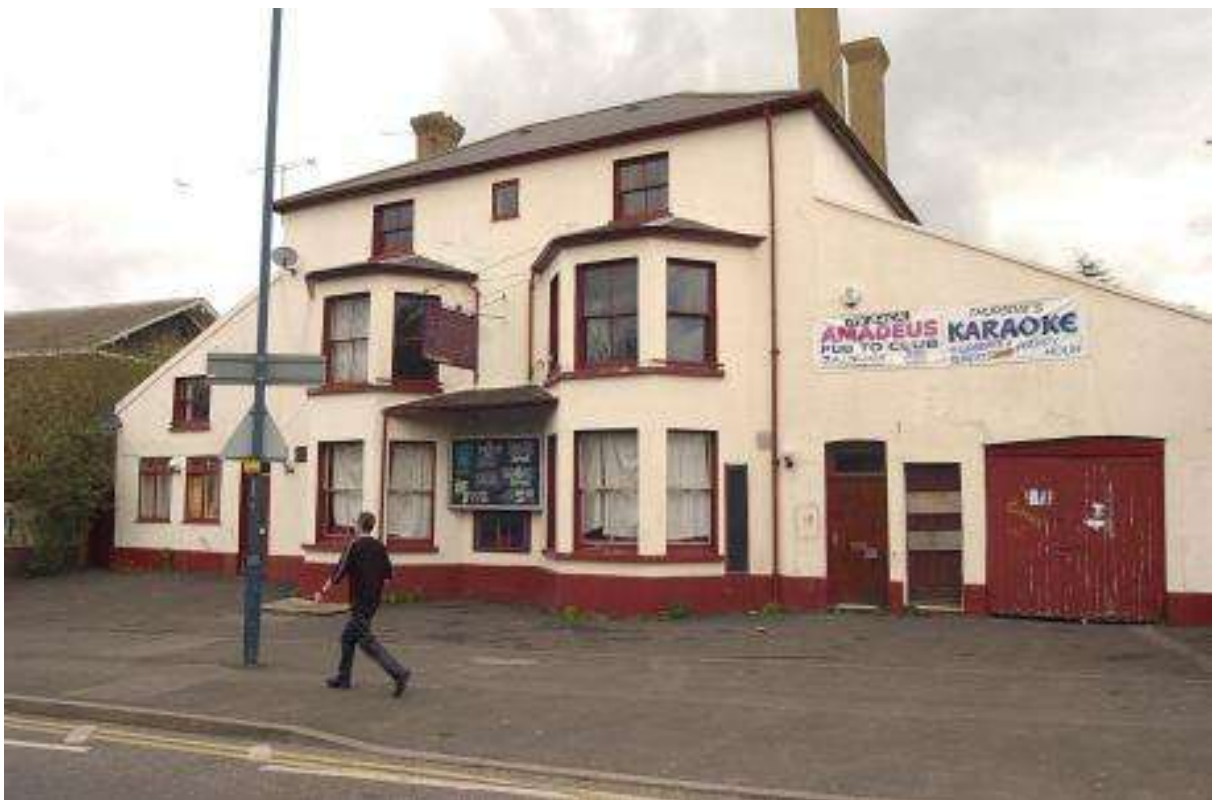
Plate 2. The site looking north prior to demolition of the public house.
